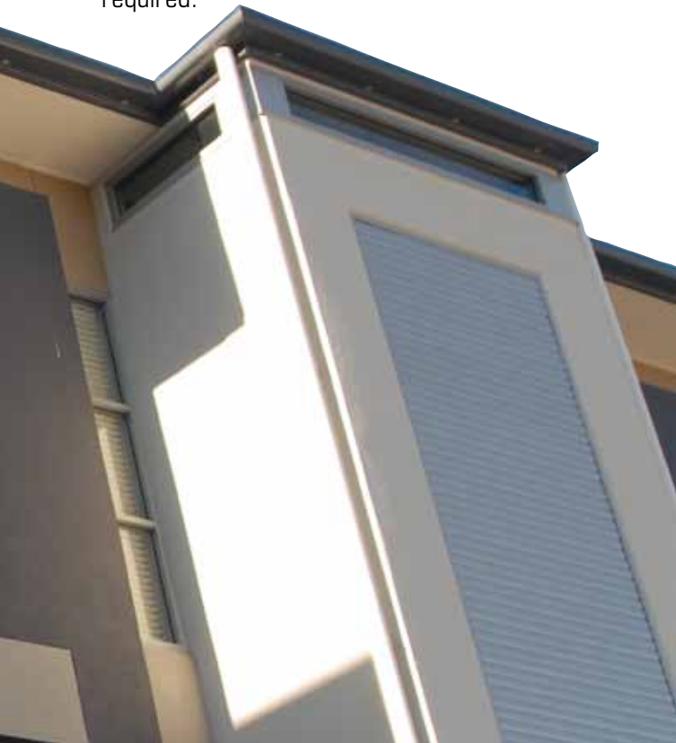
Traditional bevelback profile. Cover width 120mm
