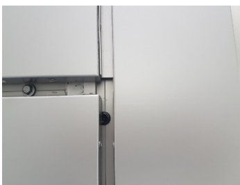
Figure 13: Vertical junction plan detail
